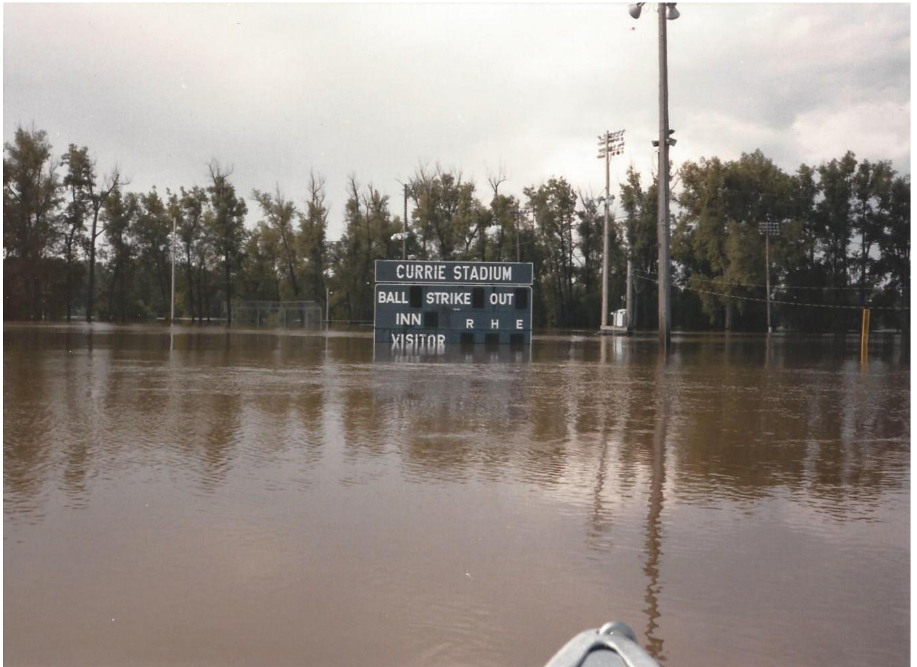
Currie Stadium experienced severe flooding during the flood of 1986.
